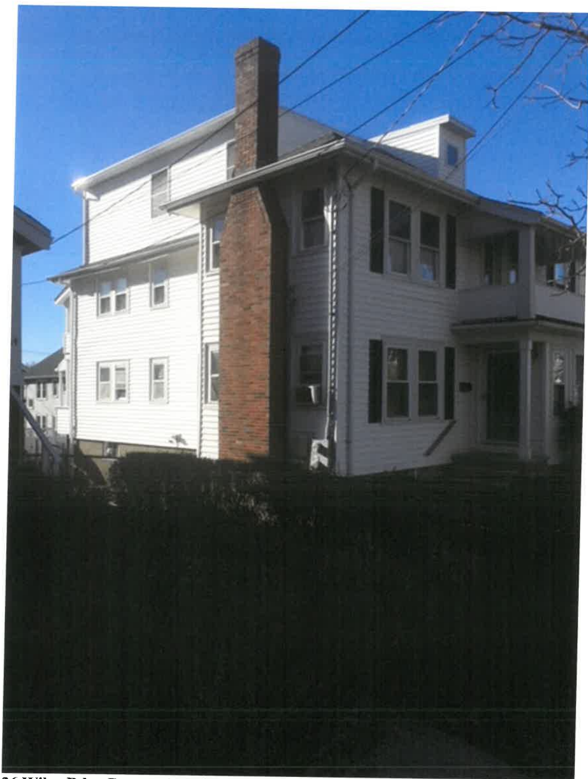
26 Wiley Rd. – Dormer & enclosed front porch. Large portion of foundation is exposed.
