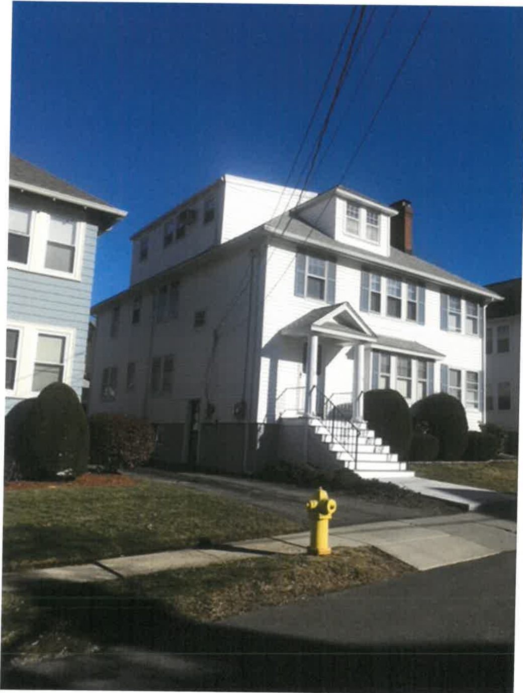
17 Holden Rd. – Dormer. Large portion of foundation is exposed.
