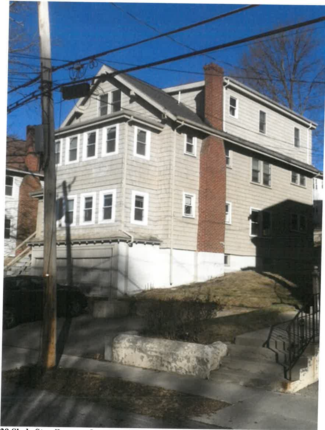
29 Slade St. – Dormer. Large portion of foundation exposed. Two-story enclosed front porch.
