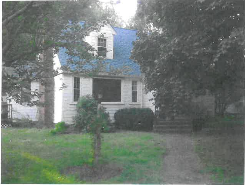
Existing Front Elevation of 136 Blanchard Road (East)
