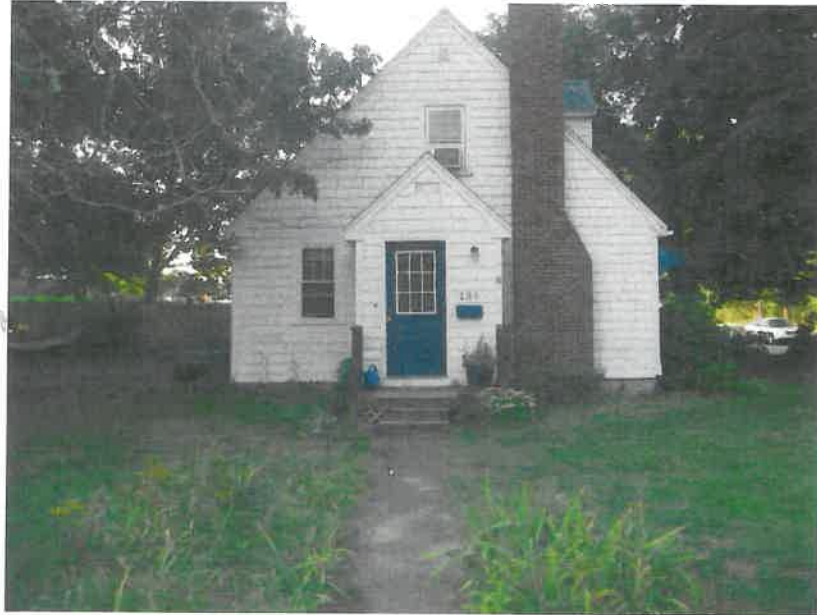
Existing Mannix Circle Side of 136 Blanchard Road (South)
