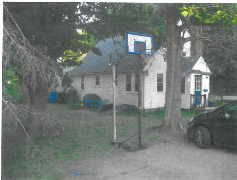
Existing Rear Elevation of 136 Blanchard Road (West)
